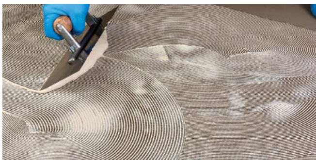
Figure 6 Spread the adhesive
