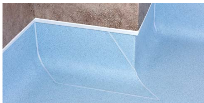
Figure 11 External corners 'wrap around method'
