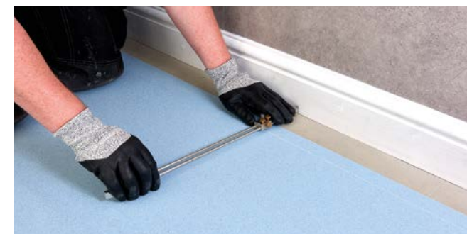
Figure 2 Scribing the wall profile
